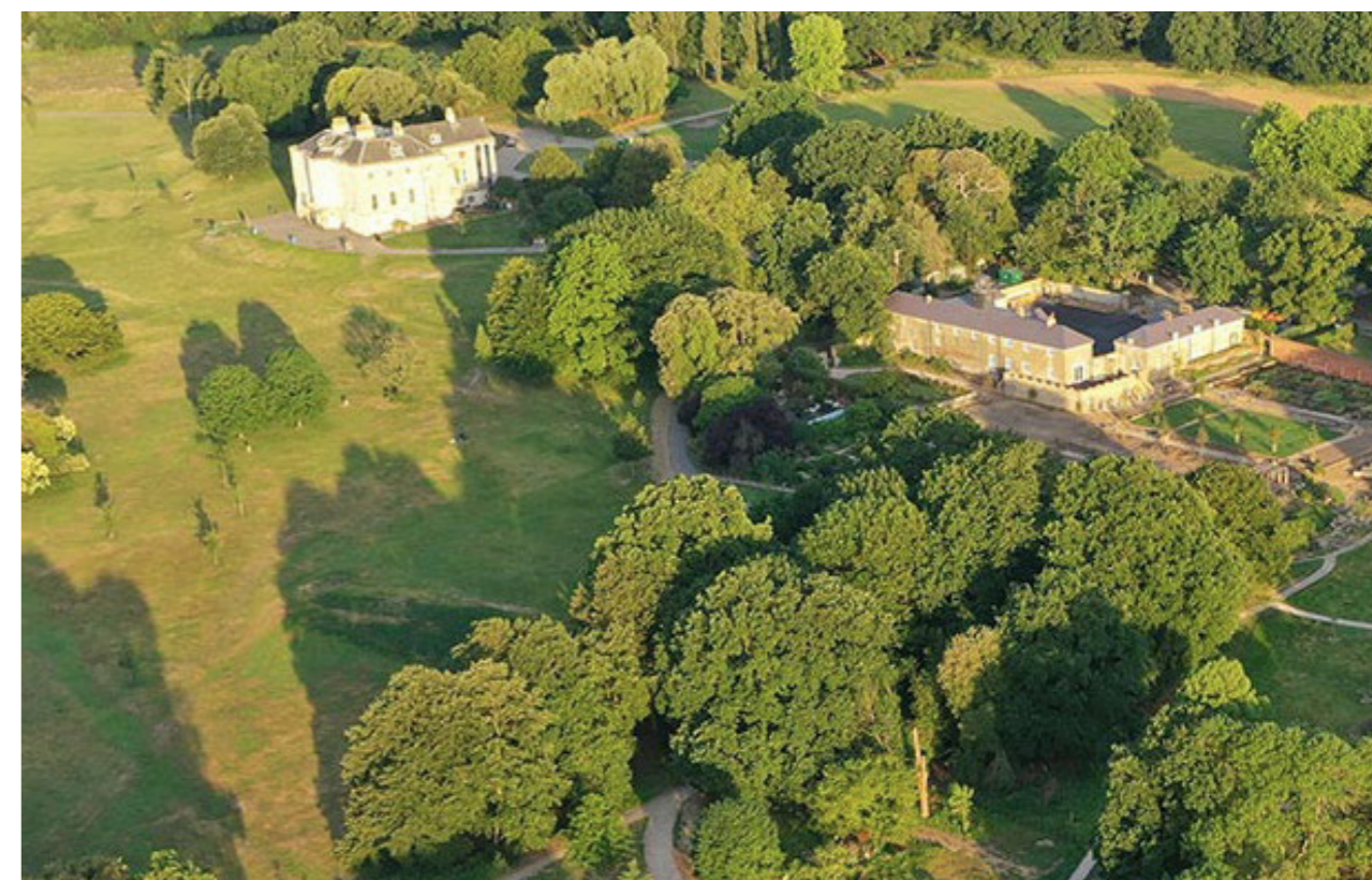
Image 2 Beckenham Place Park (photo by BDP)
